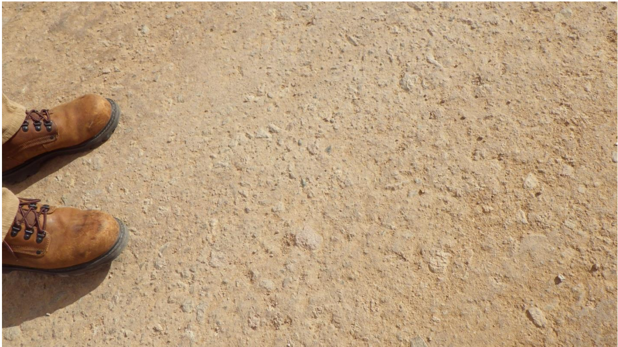
Example of the compacted surface of the road
