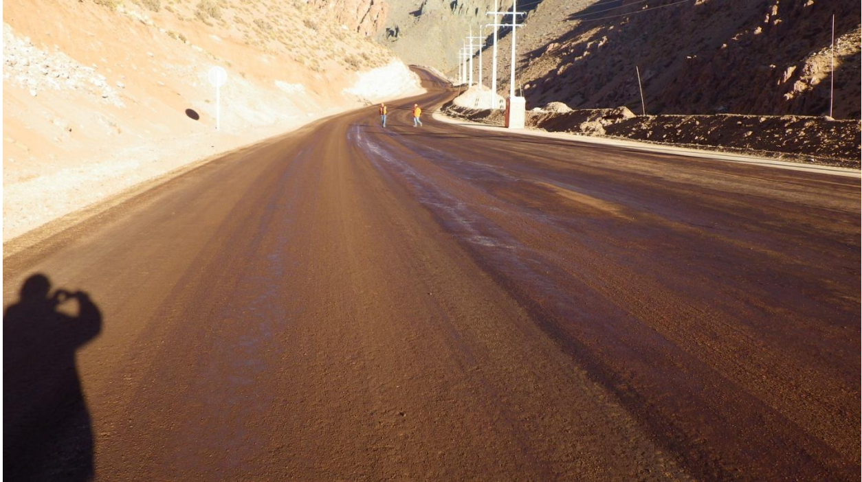
The road section after the first totes was applied (first segment)
