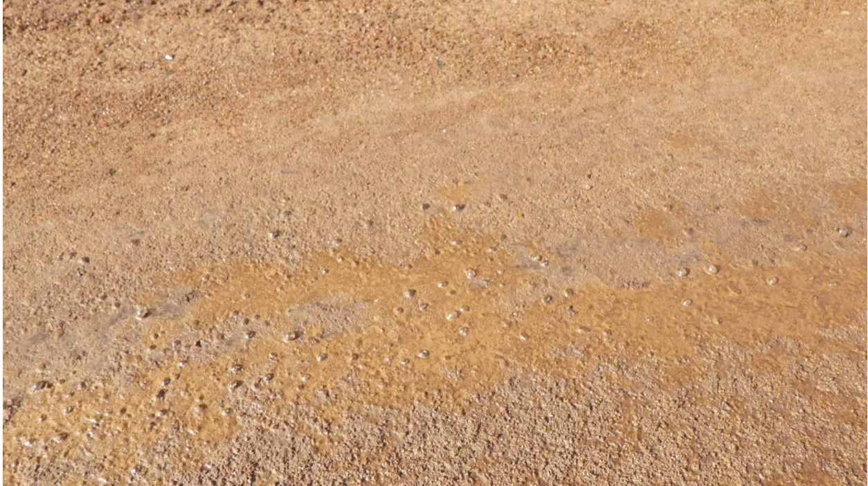
Example of how well the Earthbind 100 solution soaked into the compacted surface
