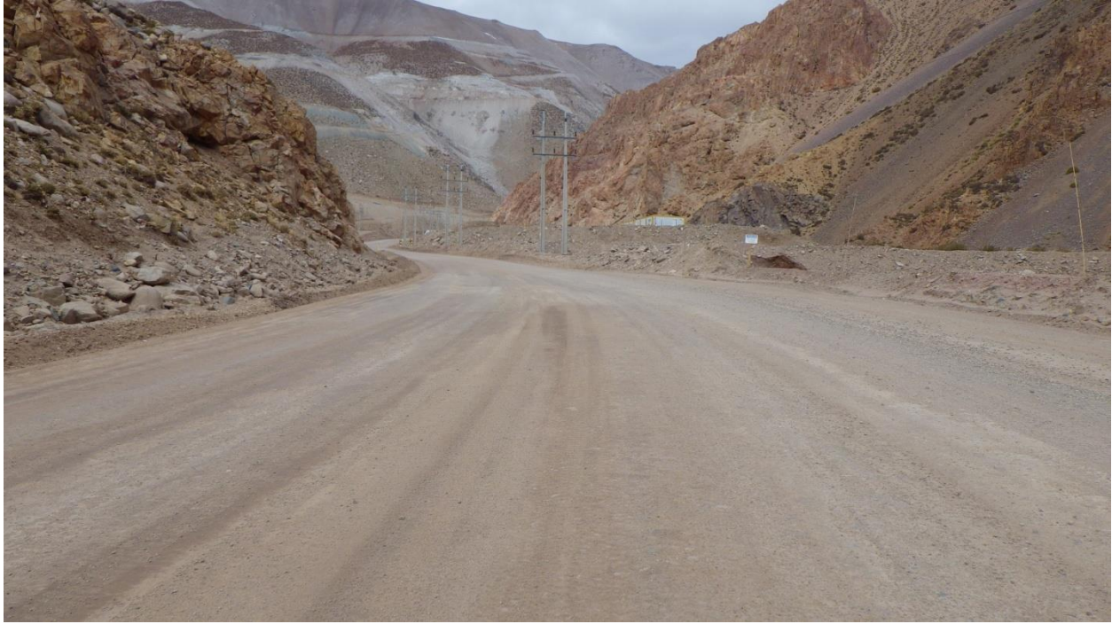
Trial road prior to application
