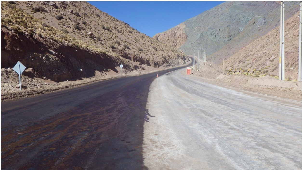
The left side of the road completed with the second tote of Earthbind. Note that the magnesium chloride crystals covered with the Earthbind solution.
