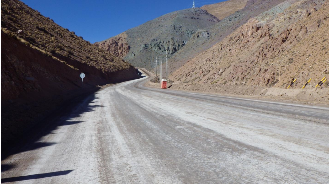
The trial road section covered with magnesium chloride crystals
