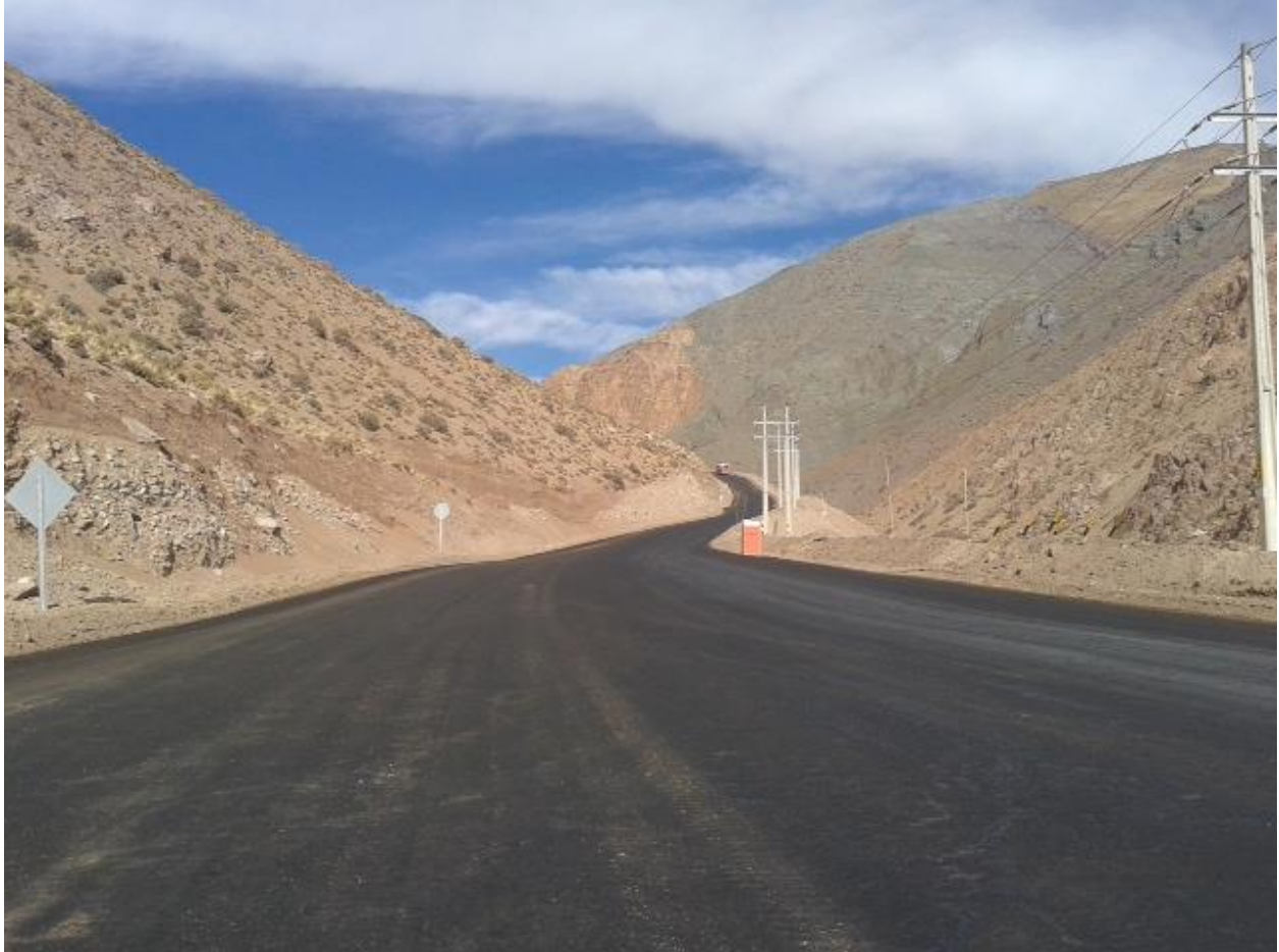
The trial road section completed.
